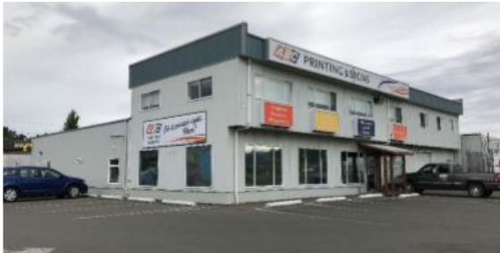
Figure 4: Existing Two-Storey Building
