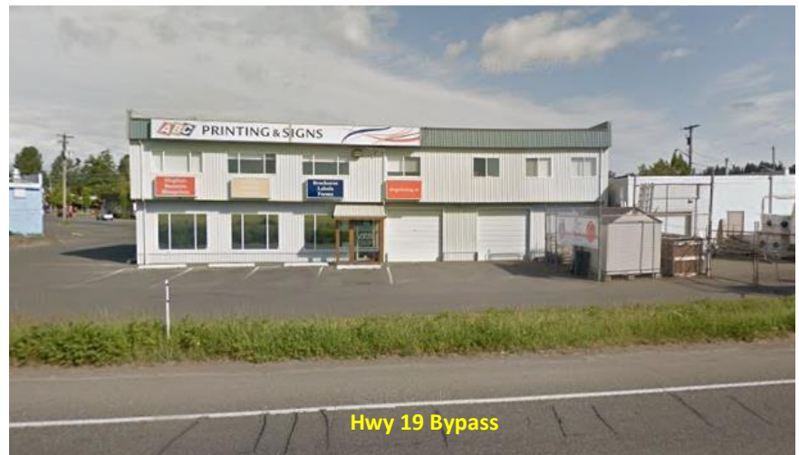
Figure 3: View of Property from Hwy 19 Bypass
