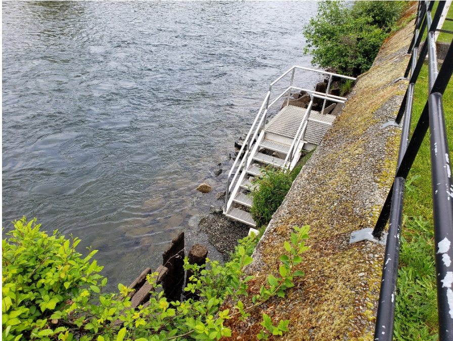
South (Downstream) Platform – May 2019
